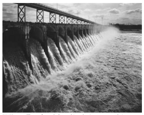
**FIGURE 11.24** The out-flow end of water-driven electric generators producing power at Wilson Dam (part of the Tennessee Valley Authority). The plant can generate electric energy at a rate of over 100,000,000 watts.
